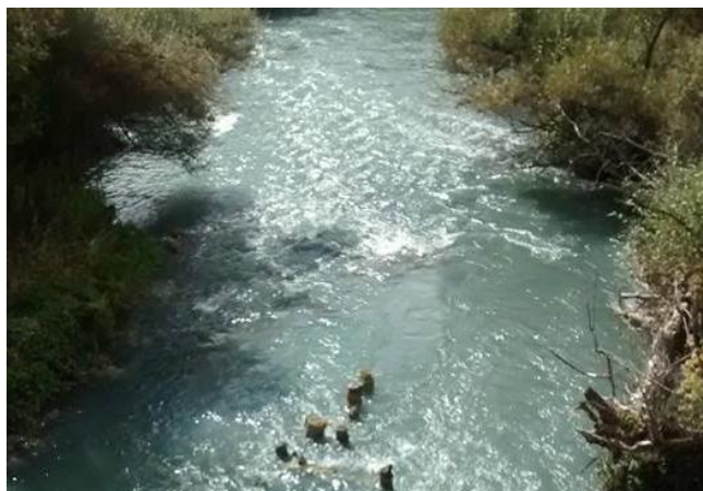
When the HPP is working
