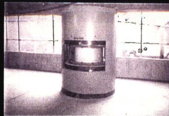
Steel Tube to Support Column Load
