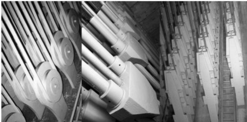
Figure 1.18 Strand anchorages: (a) parallel air-spun, (b) helical, and (c) prefabricated.
