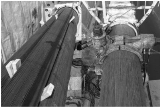
Figure 1.17 Parallel wire AS cable during wedging and compaction.
