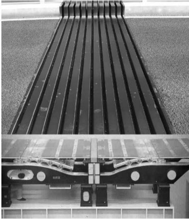
Figure 1.24 Modular and sliding plate joints.
