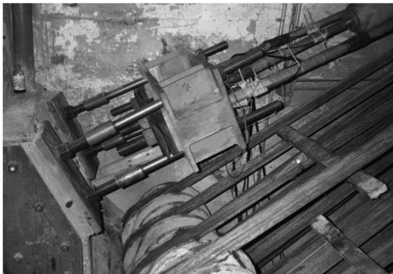
Figure 1.32 Reanchoring of a strand.
