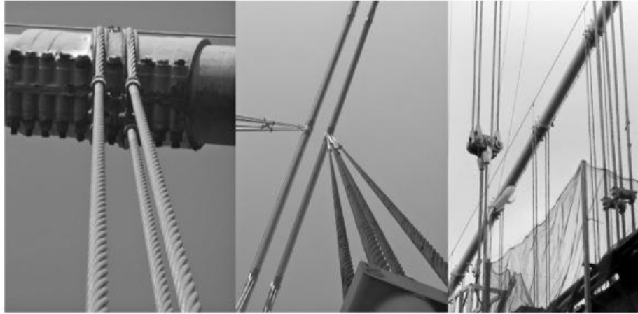
Figure 1.19 Suspenders: (a) wire rope, (b) wire ropes with spacers, and (c) wire ropes and prestressing helical strand.
