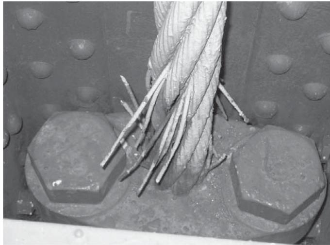
Figure 1.21 Wire breaks in suspender at the bottom socket.
