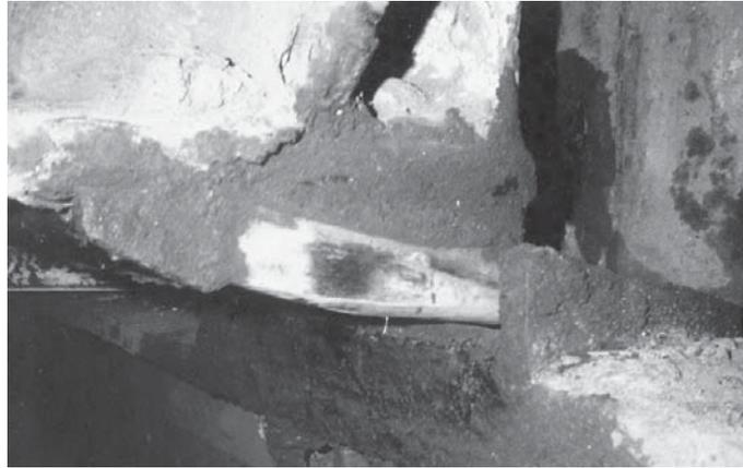
Figure 1.4 Overextended sliding bearing under the subway tracks.
