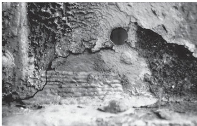
Figure 1.6 Typical crack in roadway stringer, propagating beyond a hole.
