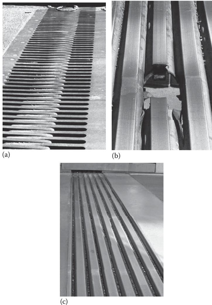
Figure 1.14 Roadway expansion joints: (a) finger, (b) modular, with broken spacer bar, and (c) new modular joint.
