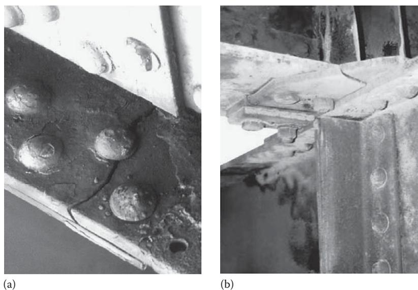
Figure 1.7 Cracks in (a) bottom chord, truss D and (b) stringer bearing.
