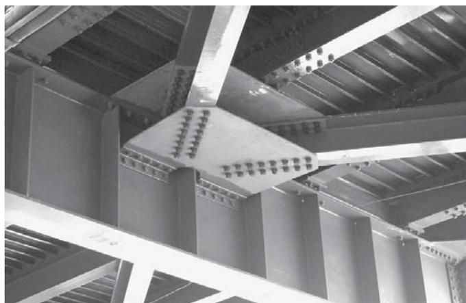
Figure 1.13 New lateral bracing under the upper roadway.
