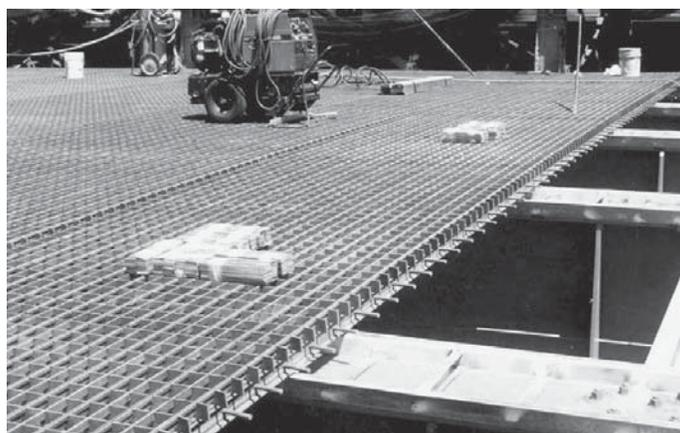
Figure 1.15 Lower roadway steel grid deck under construction.
