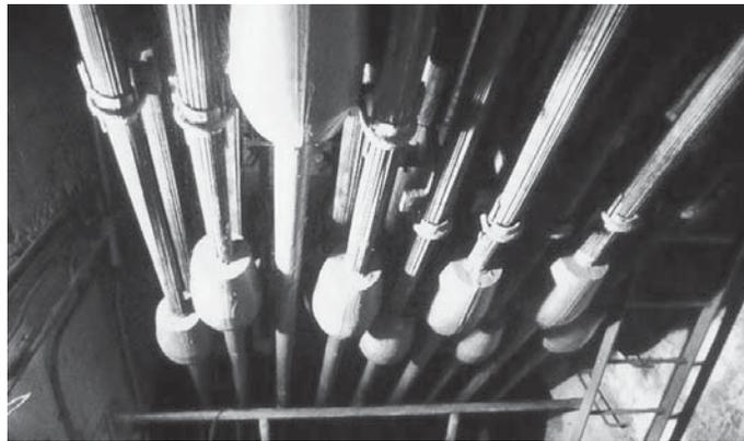
Figure 1.17 Nine transferred strands, cable C, Manhattan anchorage.
