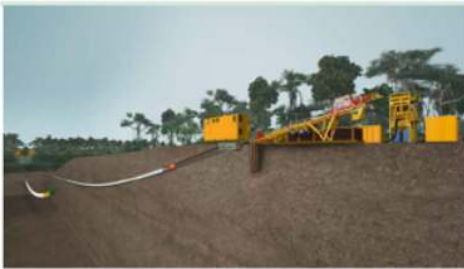
HDD RIGS: Trenchless pipeline laying
