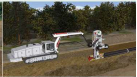
PIPE EXPRESS®: Semi-trenchless installation of pipelines
